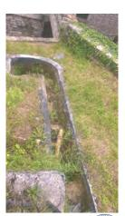
Open channel across the second garden downstream the intake, upstream (left) and downstream (right) ( $B\sim45\,\mathrm{cm},\ h\sim40\,\mathrm{cm},\ drops$  of the channel bottom  $\sim30\,\mathrm{cm}$  (1 m).
